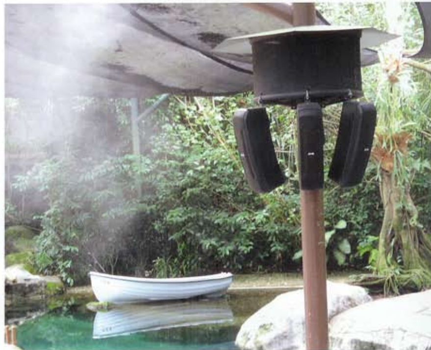
Vieta Do line loudspeakers in the Splash Amphitheatre
