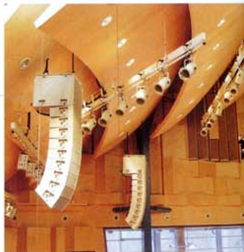
Acoustic absorption panels in the ceiling
