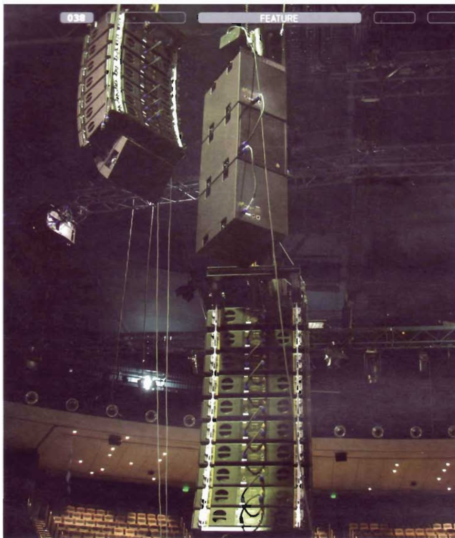
Left to right: Side hang of Adamson Y10s with underslung Spektrix downfills. Three Metrix subs lurk behind a main hang of Y10s with underslung Spektrix downfills (not visible).
